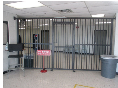
Pictured below: New security gate was added to inmate visitation.
