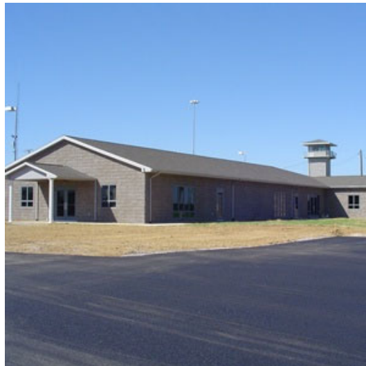
Pictured to the right: Western Region Training Center
