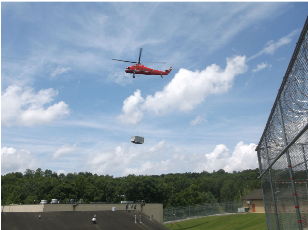
Pictured below: Helicopter moving a roof-top HVAC unit.
