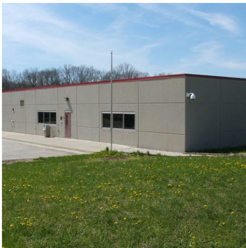
Pictured above: Eastern Region Training Center
