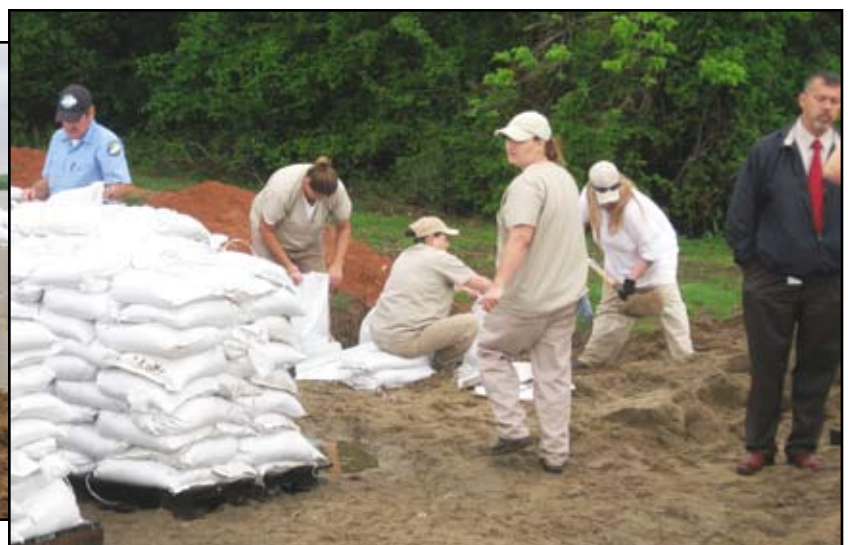
Above: KSP Inmates pitched in to help construct a sandbag wall in an attempt to protect the historic town of Smithland. KSP Inmates volunteered to fill sandbags at the prison in an effort to assist the residents of Lyon County. In one evening alone, the inmates bagged approximately 50 tons of sand in less than 2 hours for a total of 1,600 bags. Below left: KSP Deputy Wardens Alan Brown and Ernie Williams, along with Correctional Officers, supervised inmates as they assisted the residents of Smithland during the recent flooding. Below right: Western Kentucky Correctional Complex (WKCC) inmates assisted Lyon County with sandbagging efforts throughout the flooding. Pictured at far right is WKCC Warden Bryan Henson.
