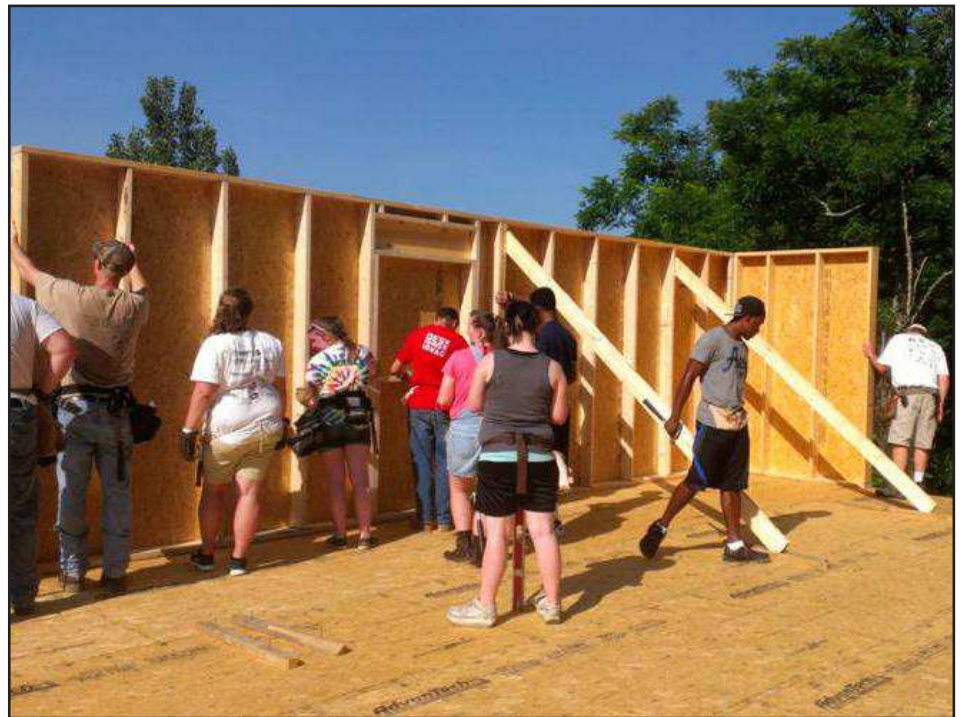
Pictured top: The Habitat for Humanity (HFH) house in Campton in the early stages. Above: Volunteers for HFH raised the walls that were constructed by inmates at Eastern Kentucky Correctional Complex. At right: Erecting the walls only took four days, compared to the weeks it would have taken if the volunteers would have had to build the walls themselves.
