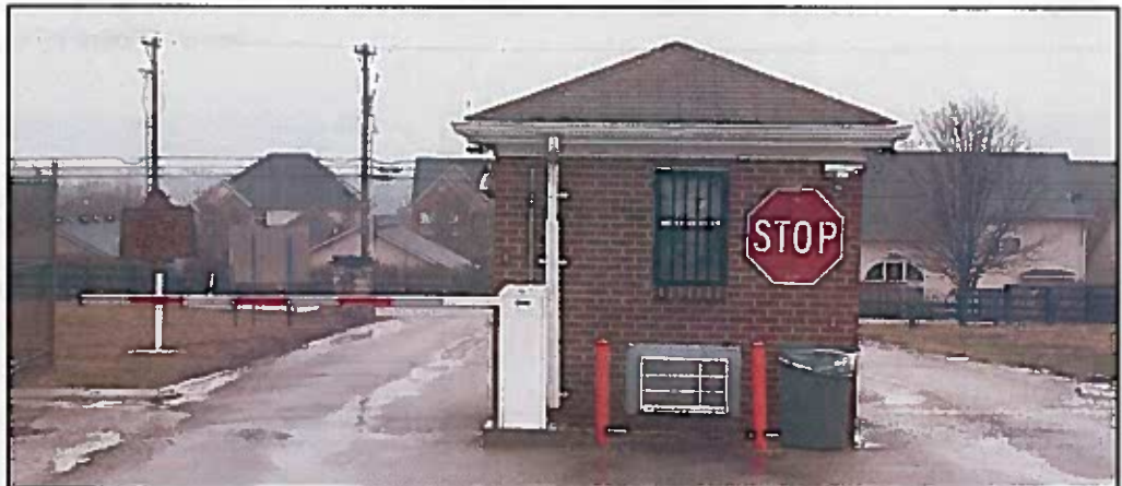
Pictured above — An electronic gate arm was installed at the main entrance of the institution.
