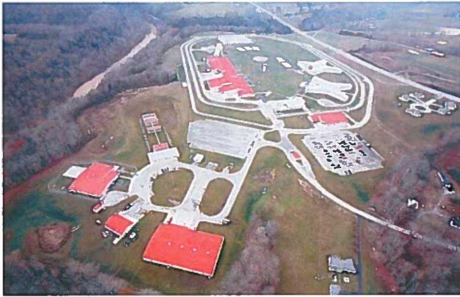
Aerial view of Little Sandy Correctional Complex.
