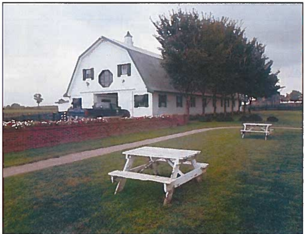
Thoroughbred Retirement Foundation Barn at BCC
