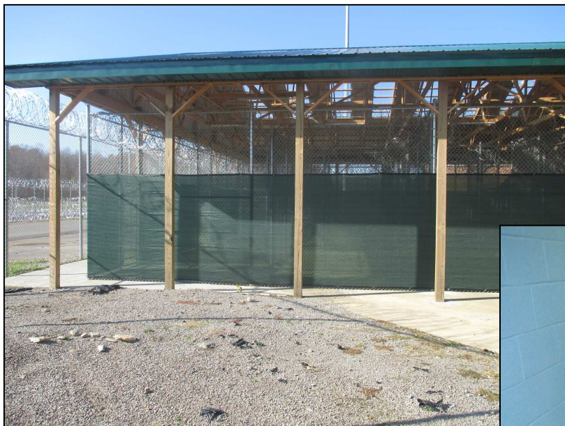
Pictured left: The bullpen fences of the Restrictive Housing Unit recreation area were covered with an industrial grade windscreen that is designed to block 88% of the wind.
