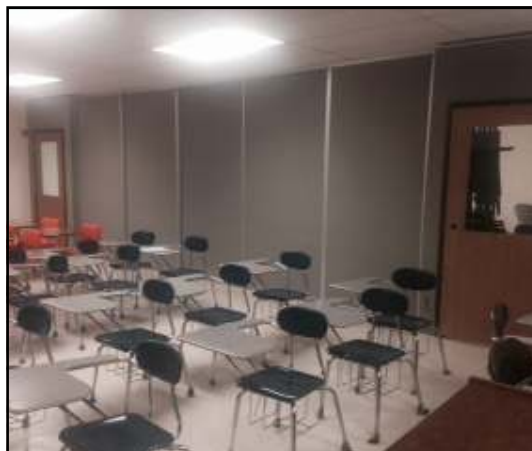
Left: Installation of a sliding panel wall in the mid-section classroom resulted in the creation of an additional classroom.
