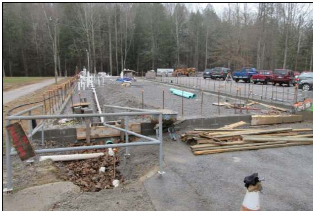
BCFC Visitation and Inmate Canteen Construction
