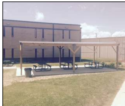
Right: Gazebos, picnic tables, and concrete pads were installed for Unit 3, Unit 4 and Unit 5.
