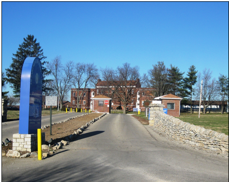
Blackburn Correctional Complex located in Lexington, Kentucky
