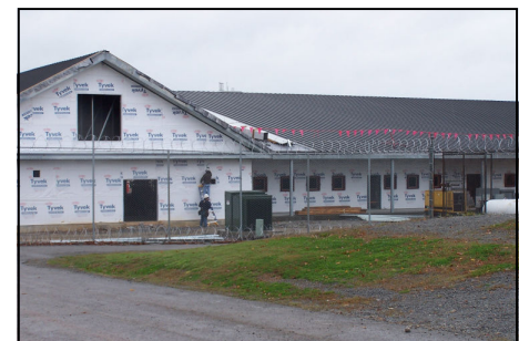
Ongoing construction of the new multi-purpose building
