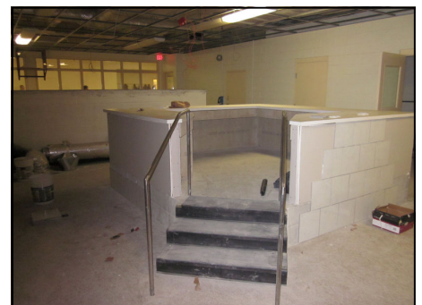
Construction on the new Medical Housing Unit
