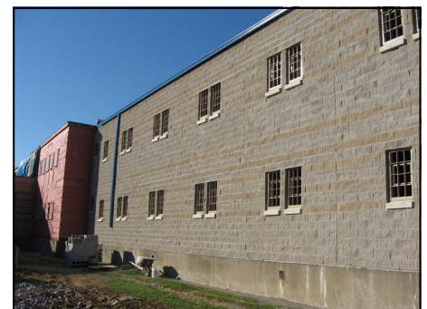
Completed renovation project on the Segregation Unit
