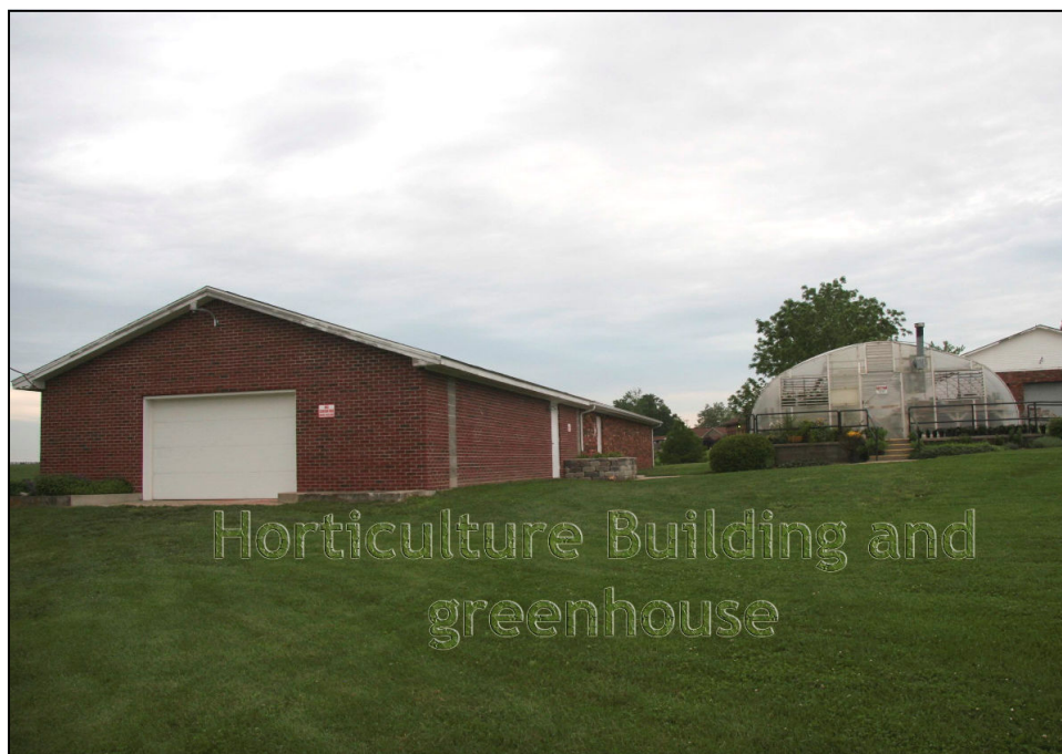
Horticulture Building and Greenhouse located at BCC
