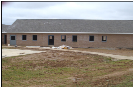
Minimum security unit - medical edition (under construction)
