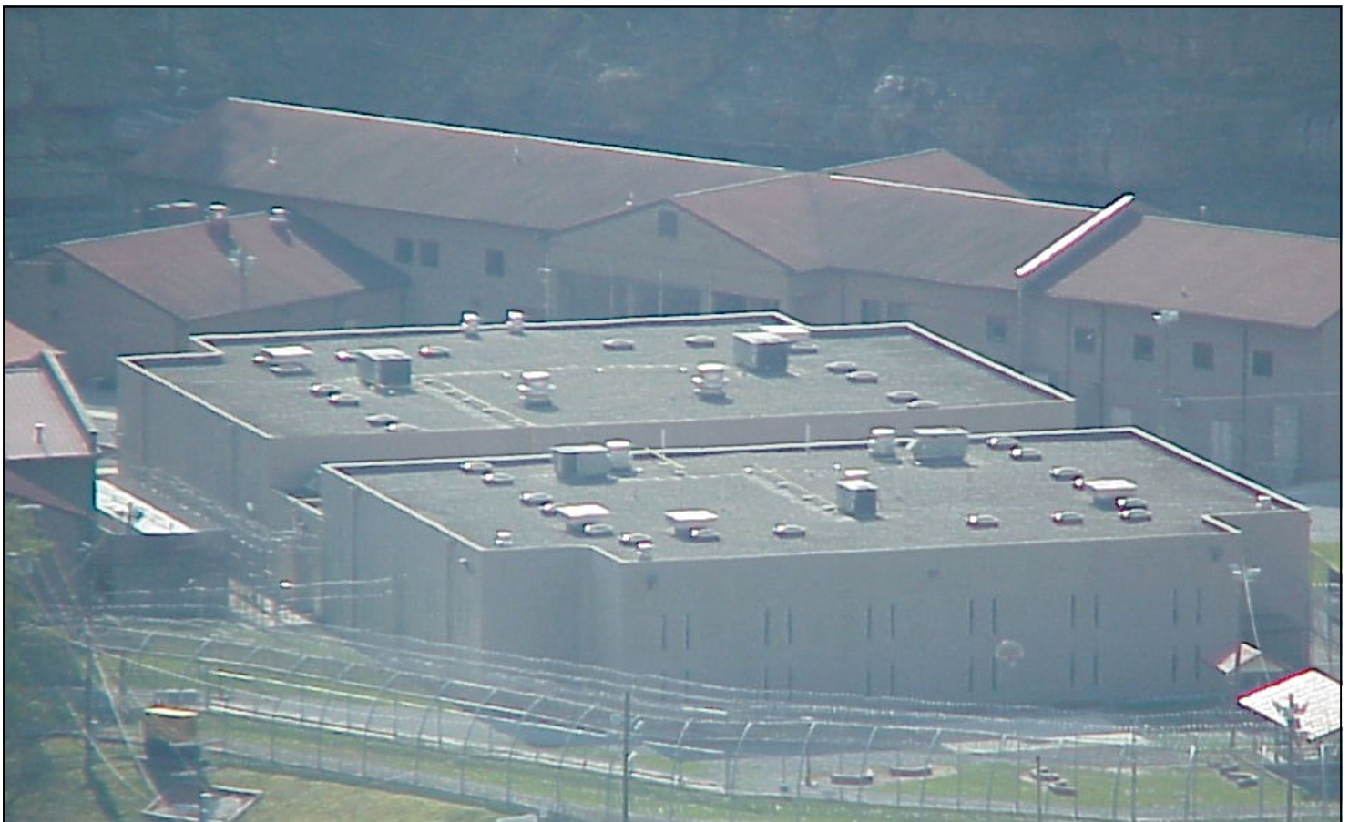
Housing Unit at Otter Creek Correctional Center
