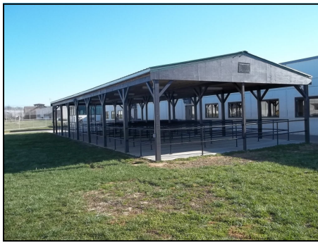
LLCC's newly constructed shelter outside the Dining Hall
