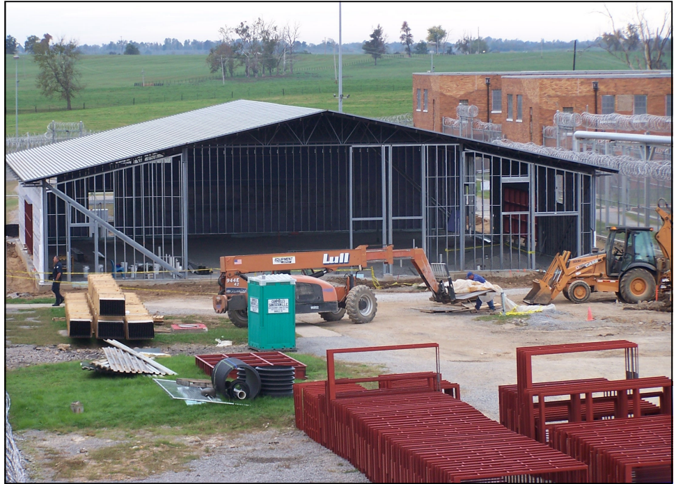
Construction continues on the new Visitation Building at NTC
