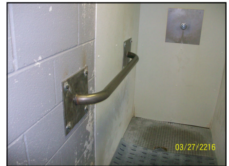
New Handrails installed in the segregation unit showers
