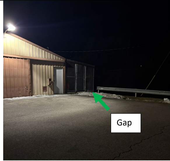
Figure 6: Gap between right front corner of Toxic building and guardrail (night). Photo taken 2/12/2026.
