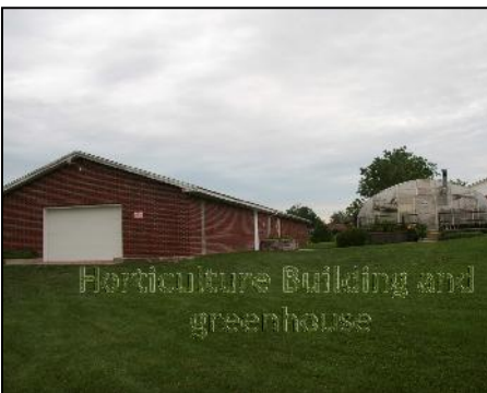
Horticulture Building and Greenhouse located at BCC
