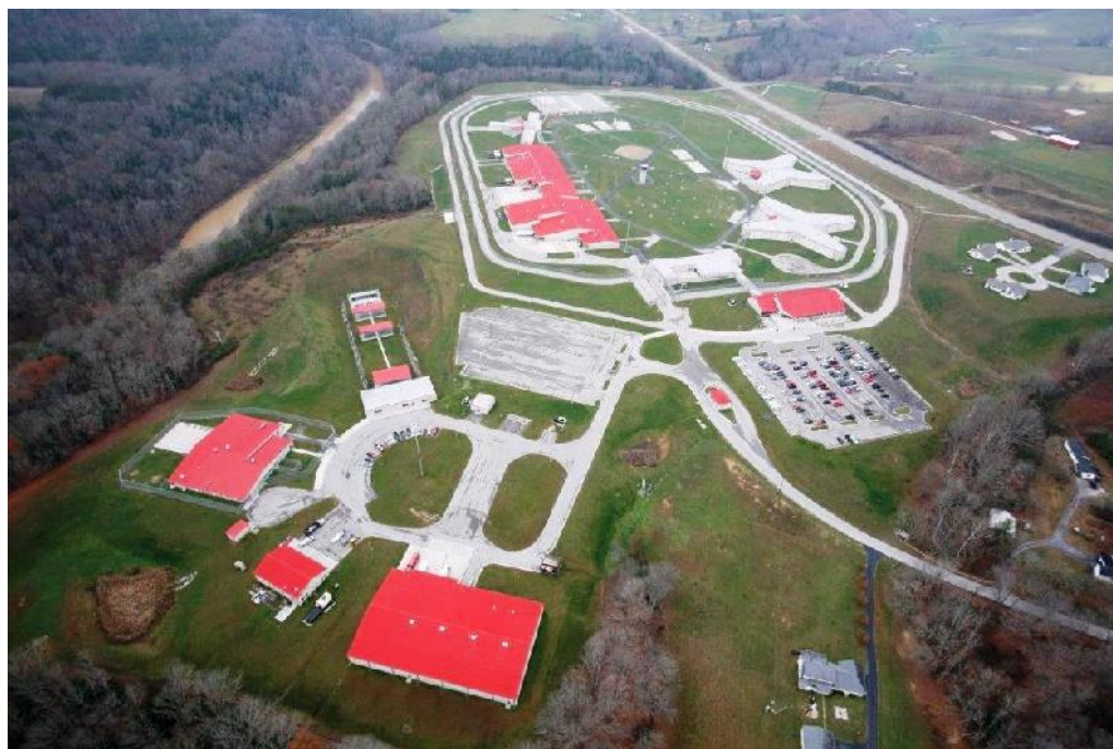
Aerial view of Little Sandy Correctional Complex
