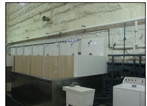
Shower renovations in 4 cellhouse
