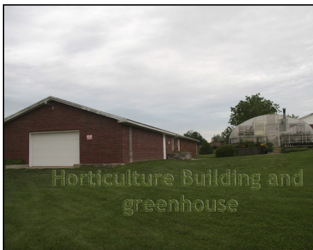
Horticulture Building and Greenhouse located at BCC
