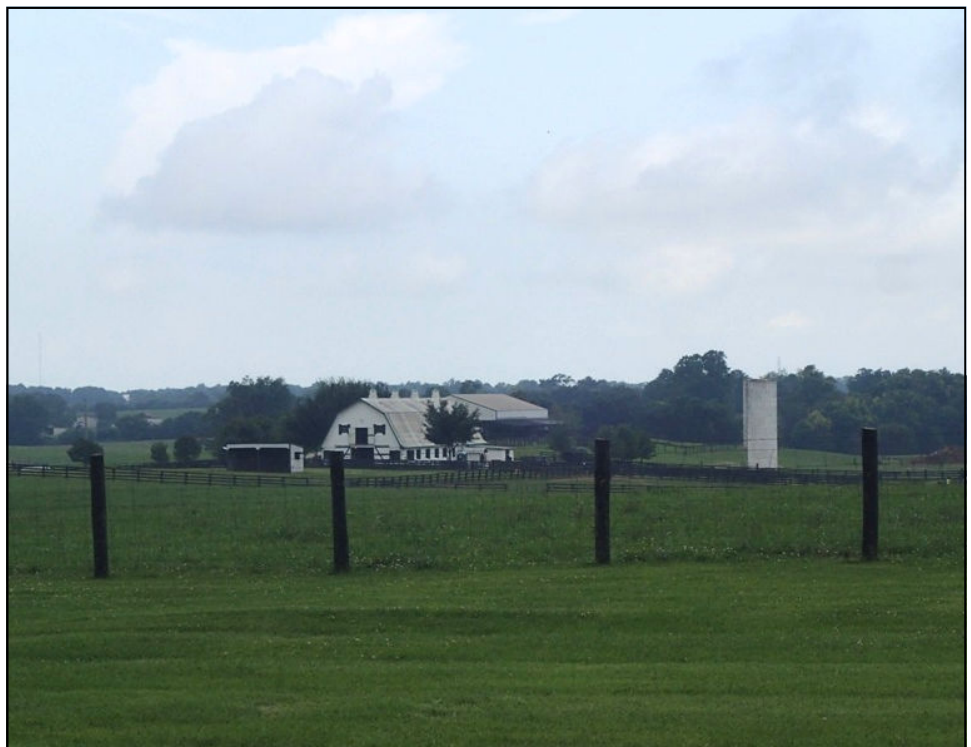
Blackburn Correctional Complex located in Lexington, Kentucky
