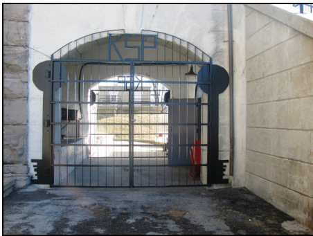
New gated entrance to Armory
