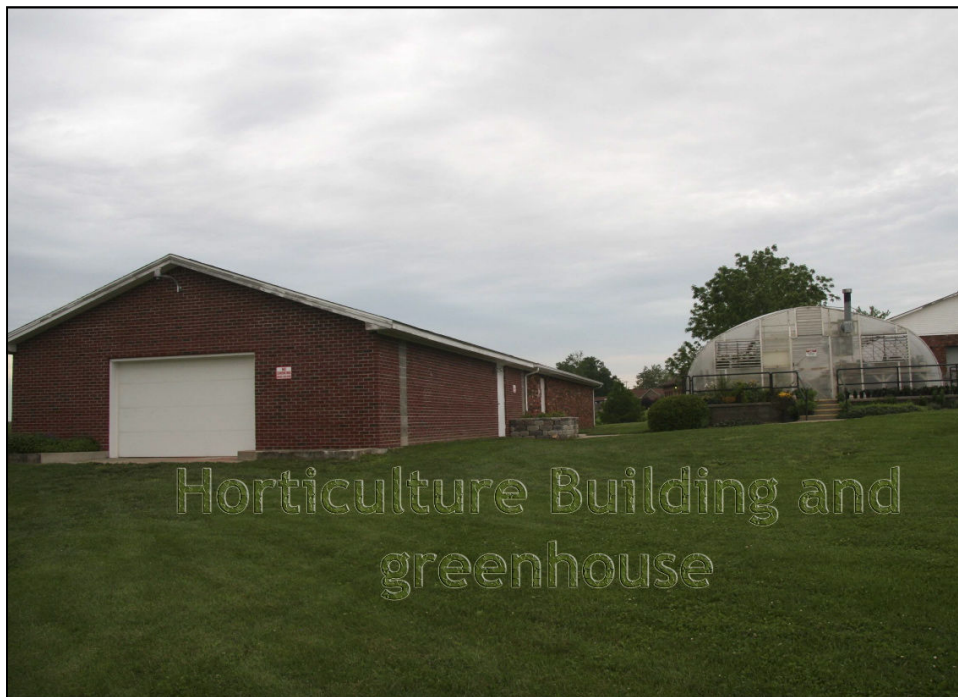
Horticulture Building and Greenhouse located at BCC
