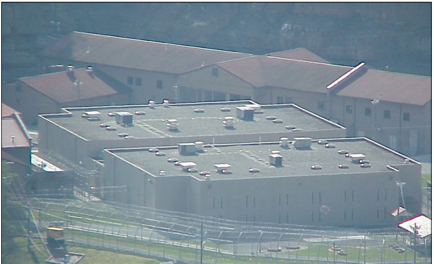
Housing Unit at Otter Creek Correctional Center
