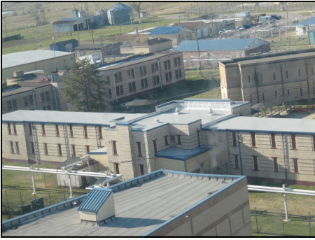
New roof on Dorm 1
