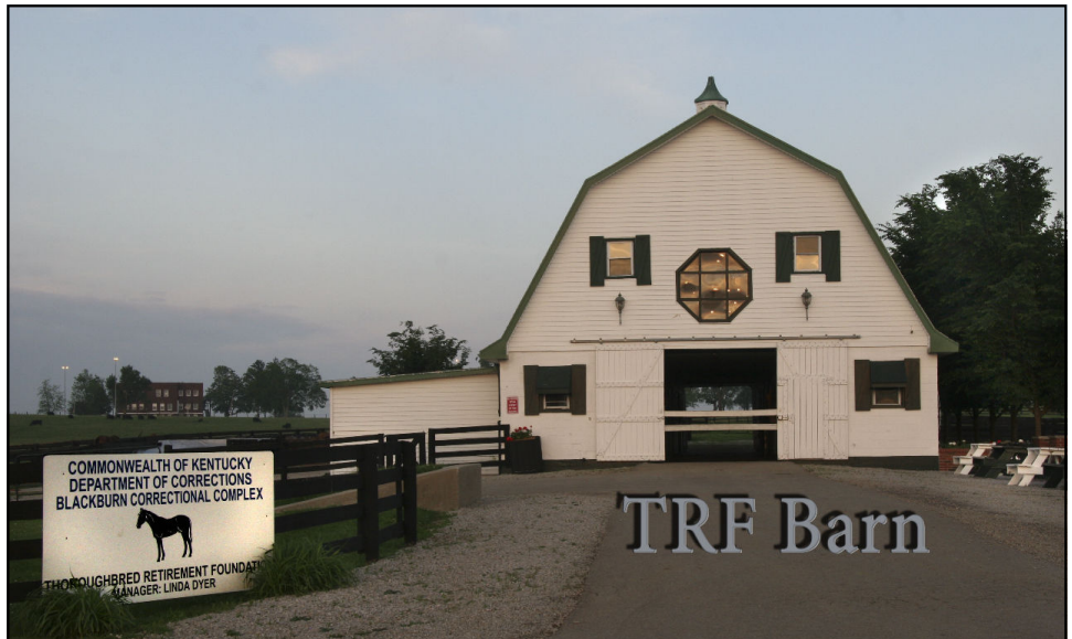
Thoroughbred Retirement Foundation Barn at BCC
