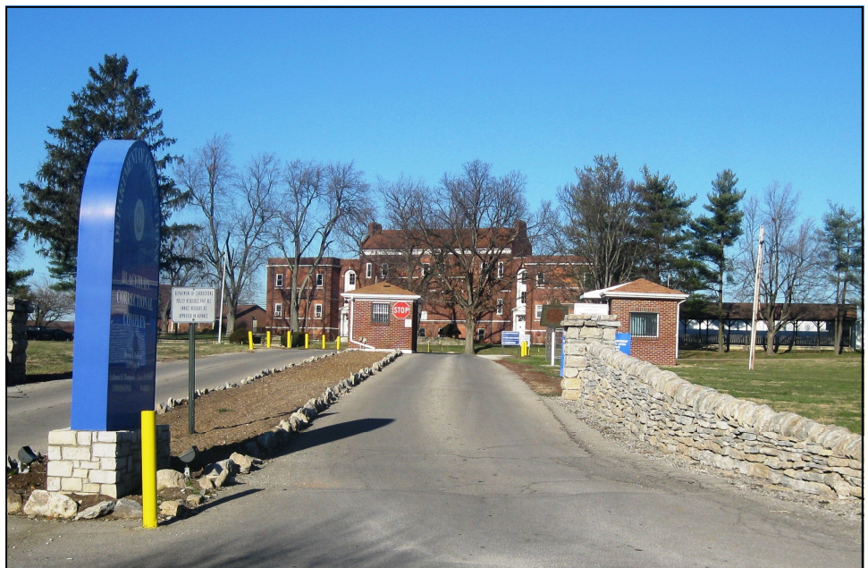
Blackburn Correctional Complex located in Lexington, Kentucky
