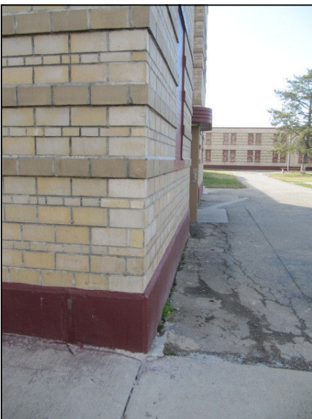
Tuck pointing of the outside walls and foundation of Dormitory 1
